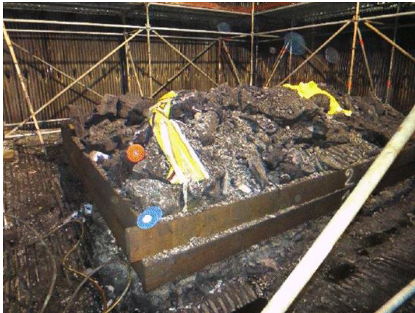
Figure 8. Cleaned floor in 2016 outage after smelt extraction but without enhanced floor washing
