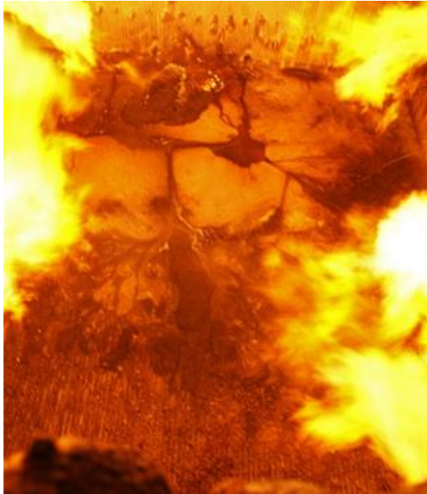
Figure 3. Floor after smelt extraction when no protection material was used, floor tubes are visible
